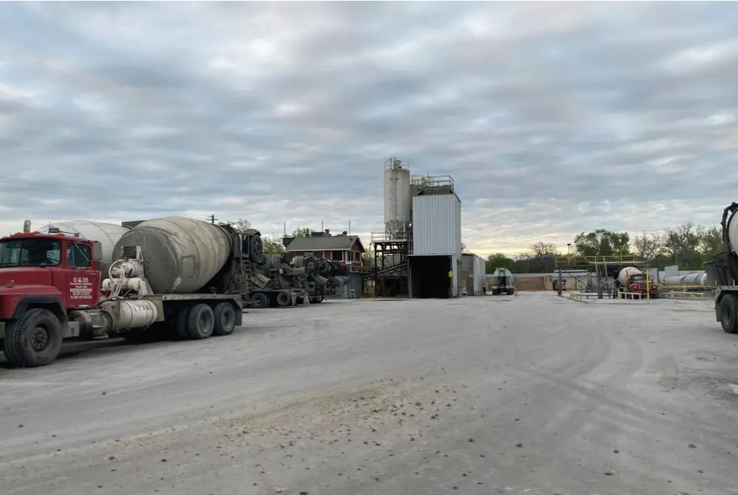
At concrete batch plants, materials like cement, sand, water, rocks, and aggregates are combined and mixed together, subsequently poured into trucks, and then transported to nearby construction projects. (Katie Watkins/Houston Public Media)
