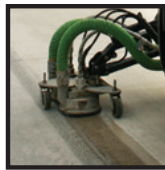
CURING COMPOUND REMOVAL
