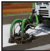
MARKING REMOVAL
