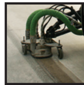
CURING COMPOUND REMOVAL
