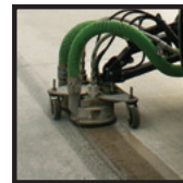
CURING COMPOUND REMOVAL
